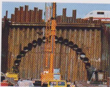
Construction of a pipe roof for a tunnel.
