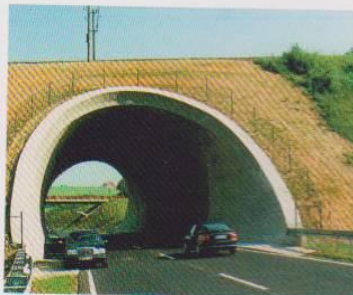
The completed tunnel underneath a railway track.
