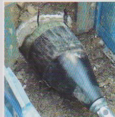
The pipe arrives at the target pit.
