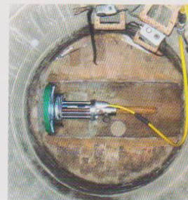
BURSTFIX 200 in the manhole
